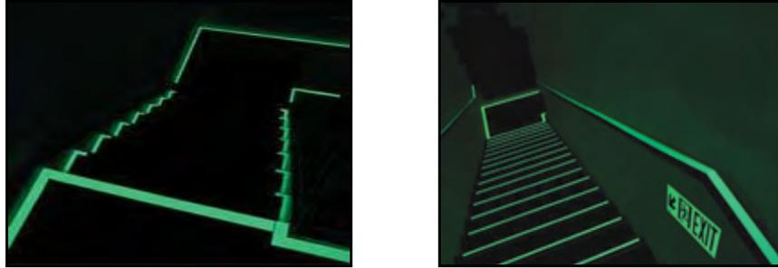
**Figure 1: Examples of photoluminescent safety marking in stairwells [4]**
